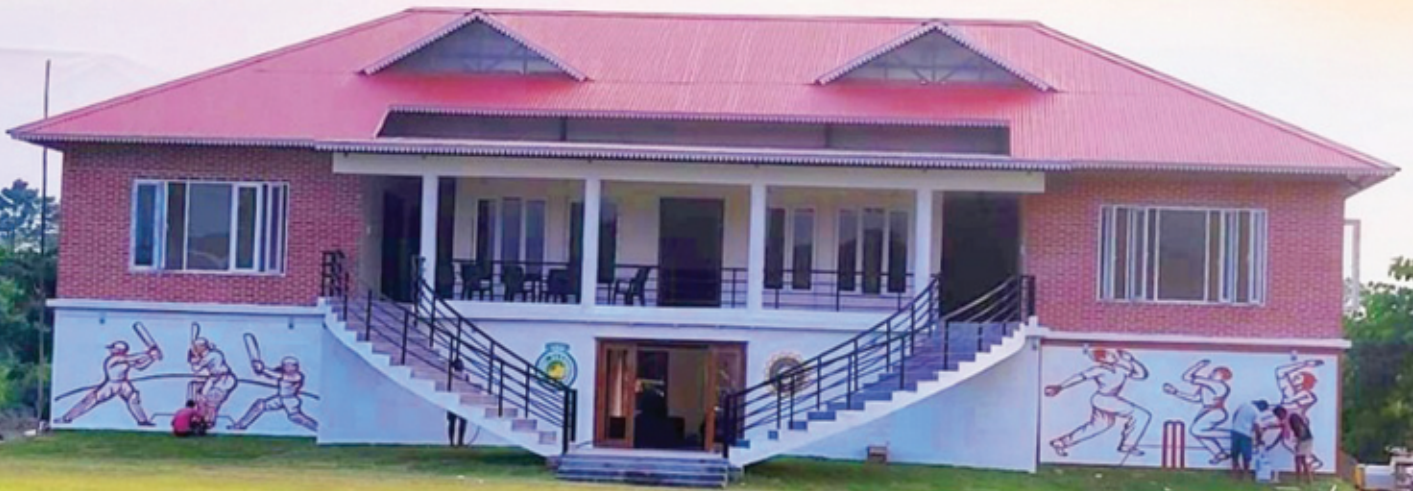
Newly constructed Amingaon Cricket Ground and Pavilion, Kumar Bhaskar Barman Khetra, Assam Cricket Association
